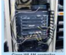
Cisco WLAN-controller
